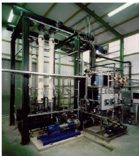
BIO LOOP at Freiburg
