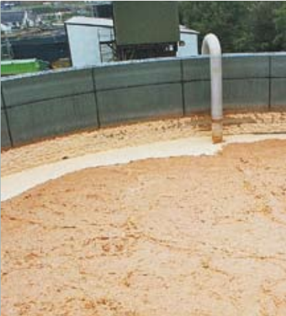
Figure 3 Aerated mixed liquor in Bioreactor
